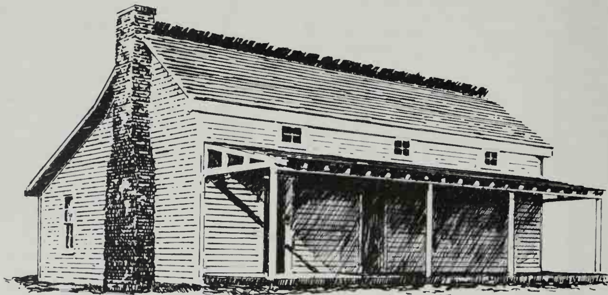
LOG HOUSE WITH CLAPBOARD SIDING
